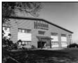
Hardinge United Kingdom facility Exeter, England
